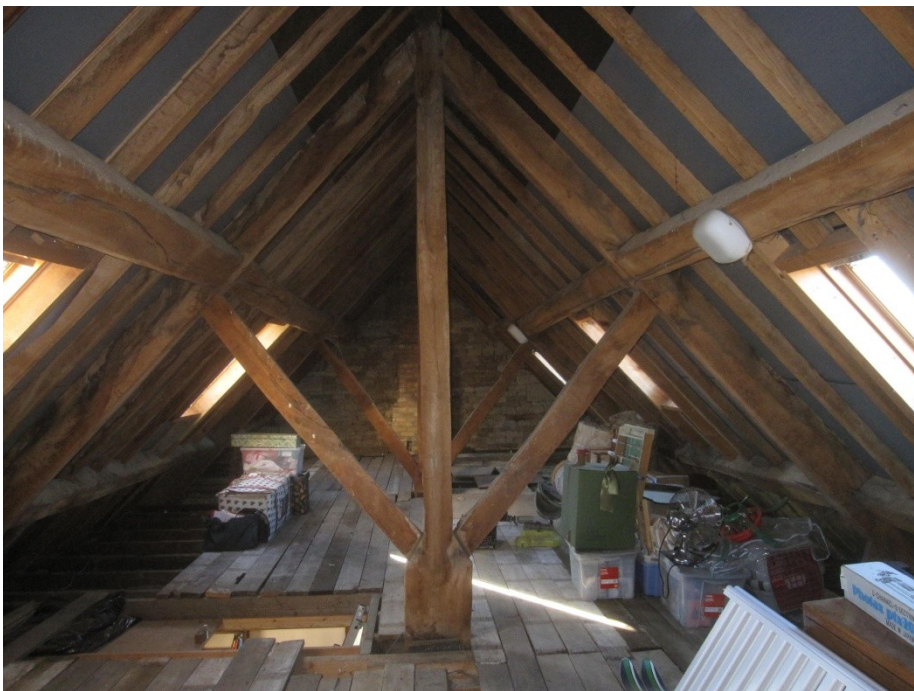
The king post roof structure, looking south
