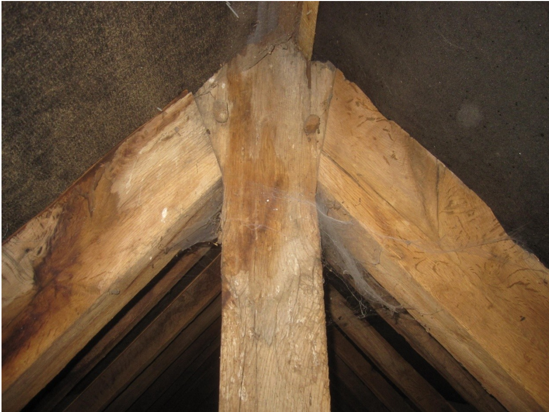
Apex of king post truss
